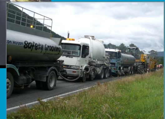
Alpine SH with freeze / thaw distress
