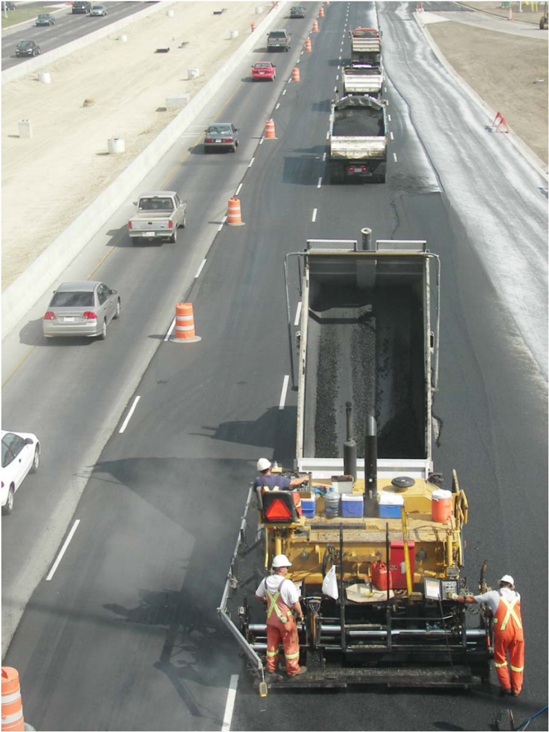
Lafarge Western Canada – Project ASM&RAP
