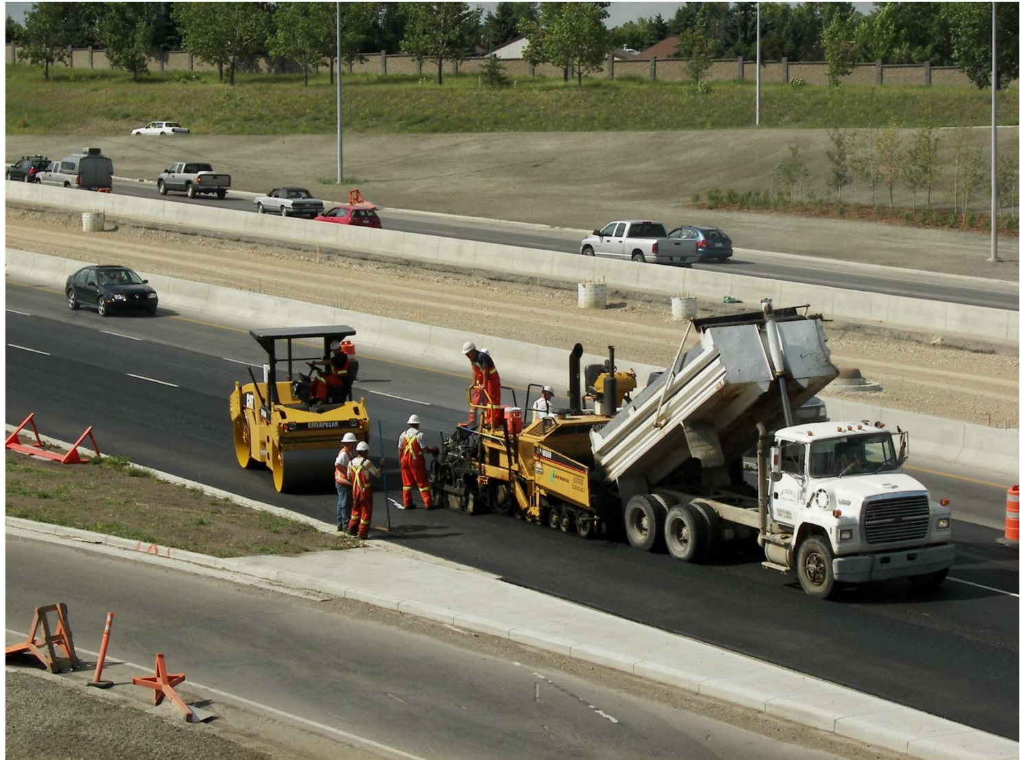
Lafarge Western Canada – Project ASM&RAP
