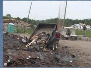
Ref: Krivit, D. (2007). Recycling Tear-Off Asphalt Shingles: Best Practices Guide . The Construction Materials Recycling Association
